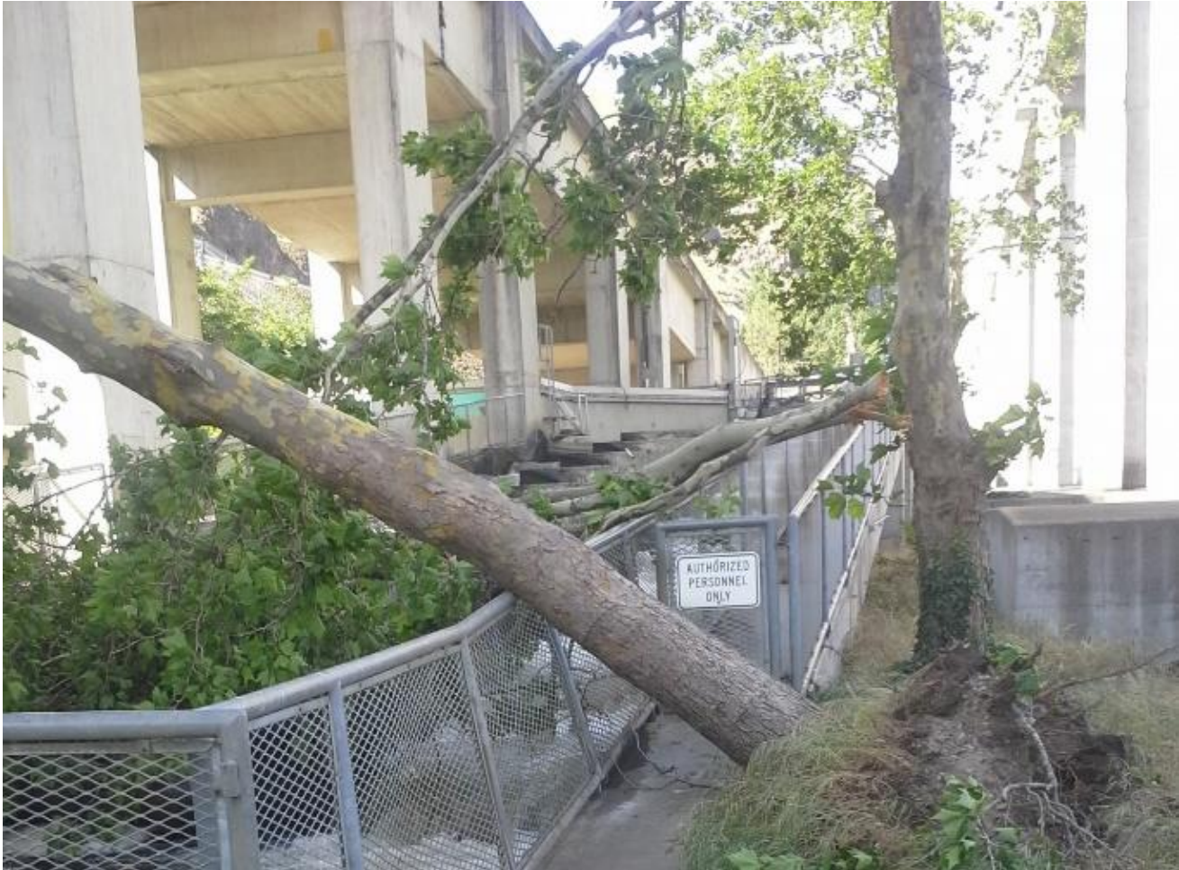
One of many trees toppled by a windstorm at the John Day project on May 30, 2020. This tree fell across the south fish ladder. No structural damage to the ladder occurred and the tree was promptly removed.
